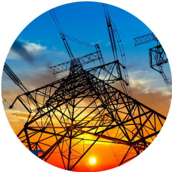
Power Generation & Transmission
